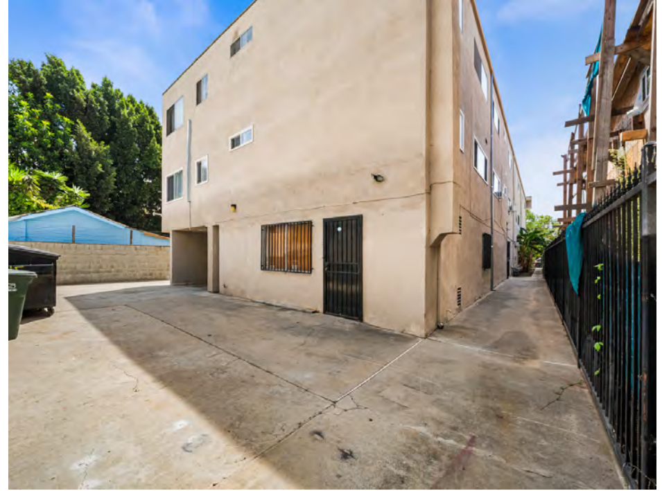
Back of Property & Storage/Bonus Room on Right
